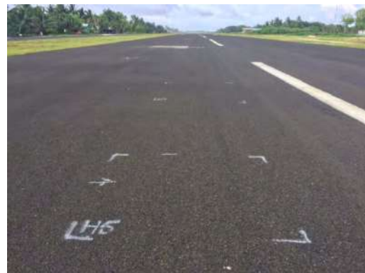
Pavement venting areas marked up. Patches were also inventoried.
